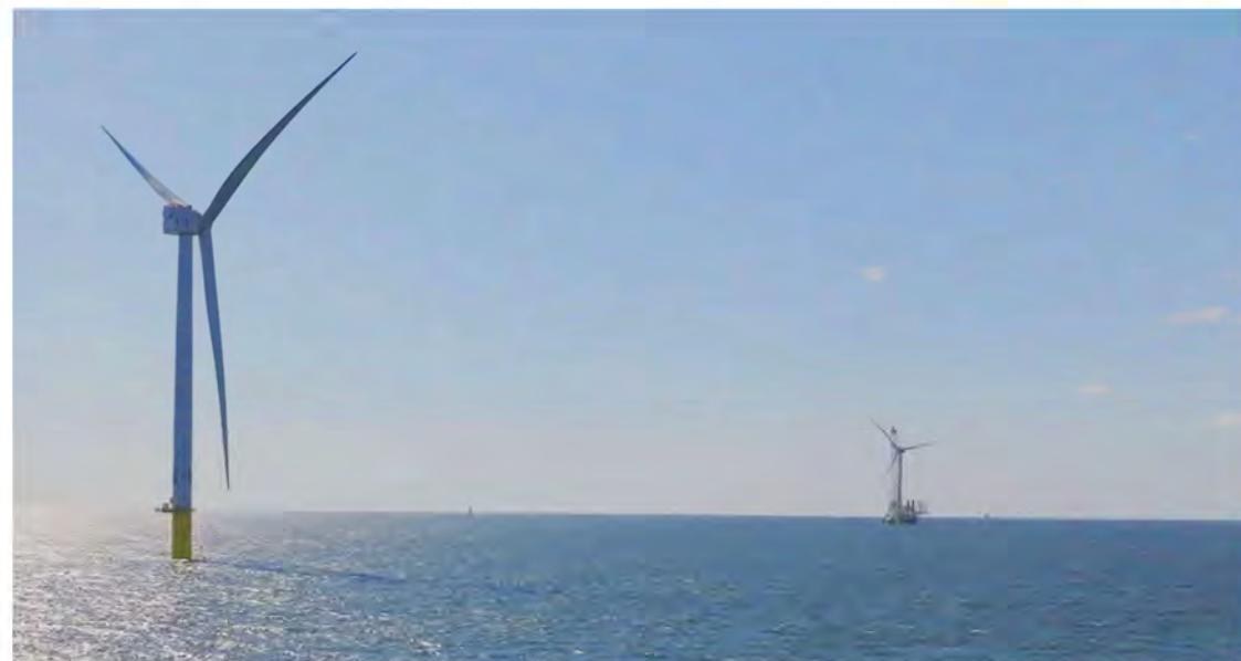
GE Haliade-X Turbines stand in the Vineyard Wind 1 Project Area south of Martha's Vineyard.
